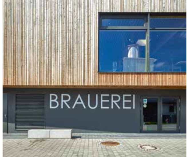
You can literally read on the facade what hides behind it.
