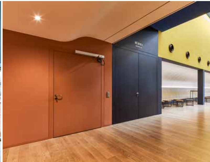
Some doors with an unusual width have an automatic closing system.
