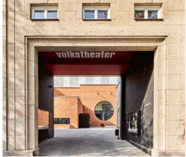
Insight: An entrance to the inner courtyard leads through the historic building stock.
