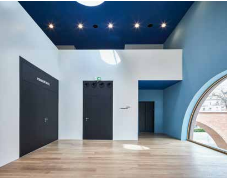
Ventilation outlets are integrated into the design of the transom panel.
