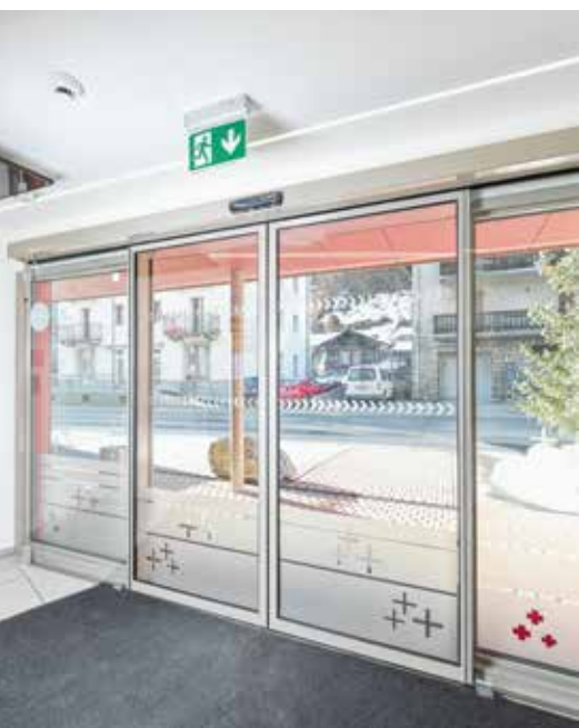
Main entrance: automatic sliding door.
