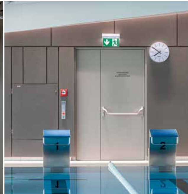
Two push bars are used for double-leaf doors. If a side element is not relevant for the required passage dimension, one handle is sufficient.
