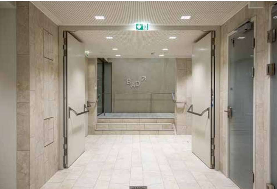
Two push bars are used for double-leaf doors. If a side element is not relevant for the required passage dimension, one handle is sufficient.
