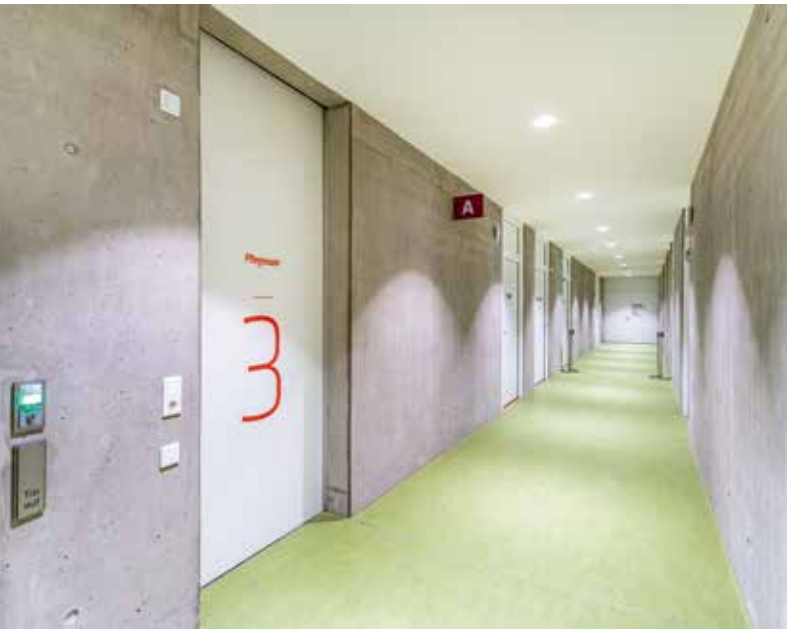
Some of the doors are room-high or have a transom panel.
