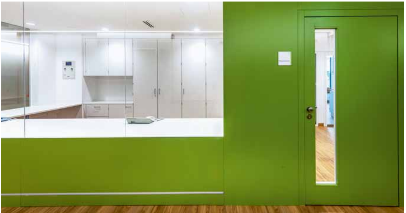
Central areas are in a contrasting colour, like here in the ward's care support post. The glazing cut-out guarantees collision-free opening of the door.
