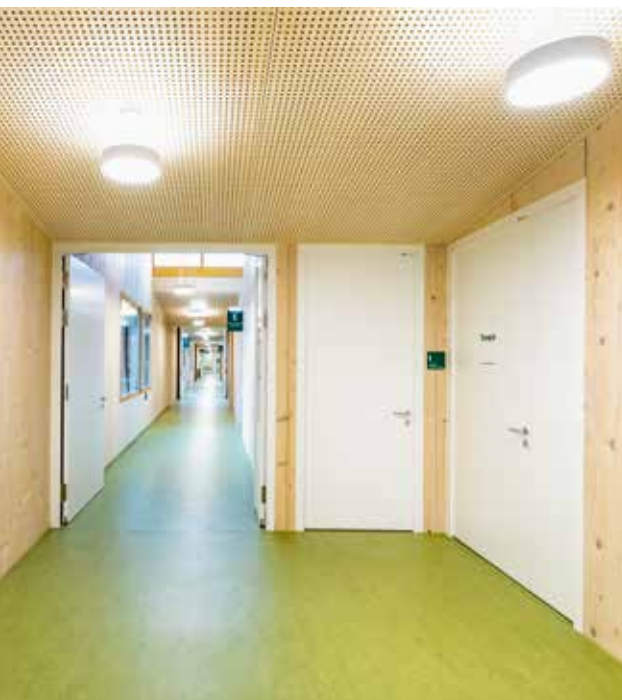
Double-leaf doors divide the corridor into sections.
