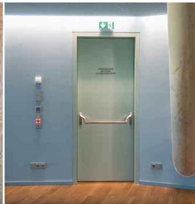
Featuring multiple escape door labels.
