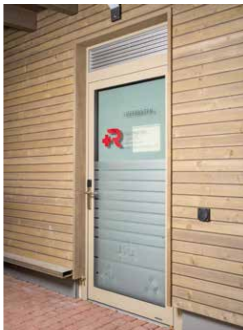
Damp room: transom panel as ventilation grille.
