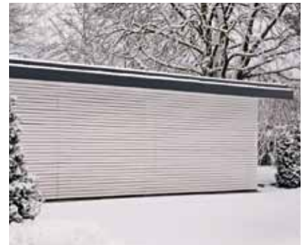
The garage doors are flush-fitted into the white timber lagging and thus barely visible.
