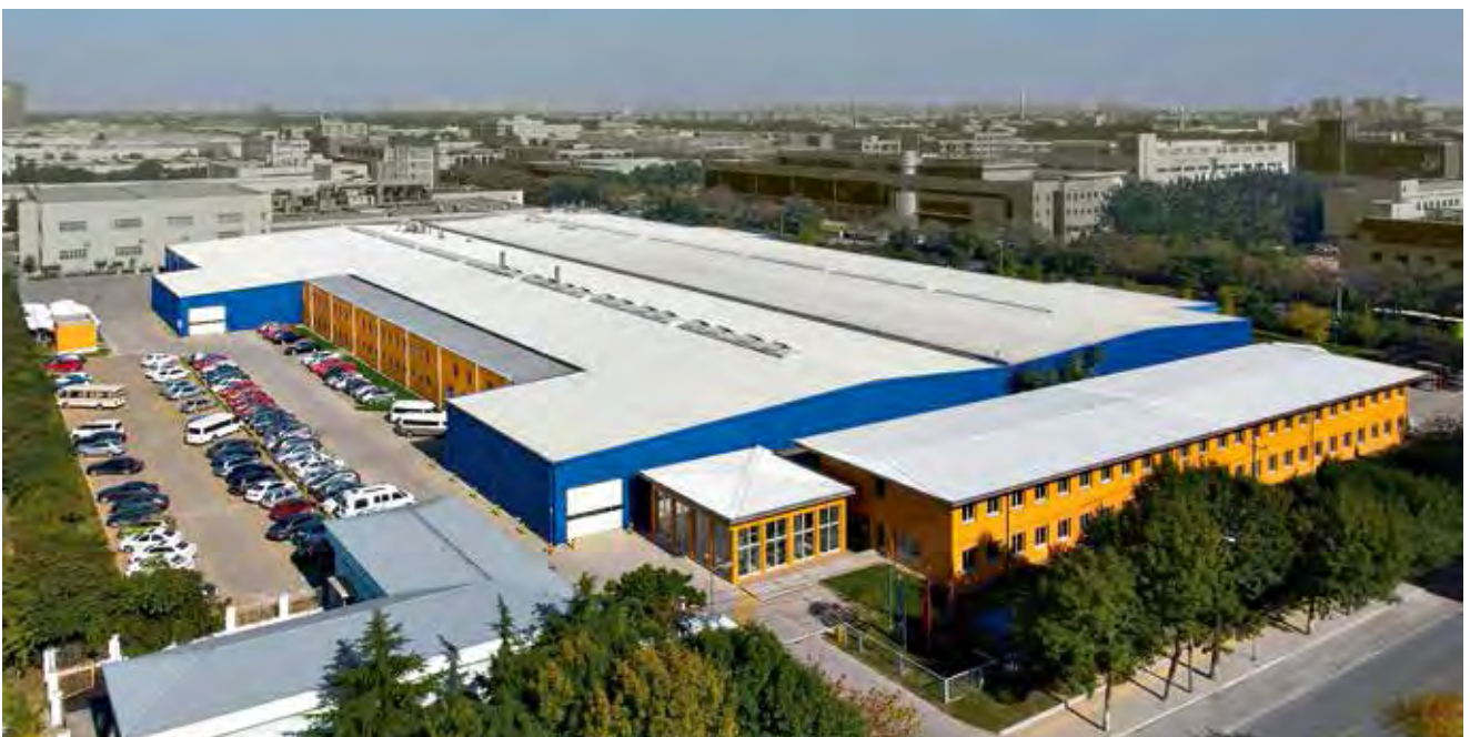
Eye-catcher: The Hörmann factory in Beijing contrasts with its surroundings.
