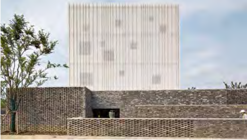
Greyish bricks – a material typical for the region – are also used for the base of the chapel.
