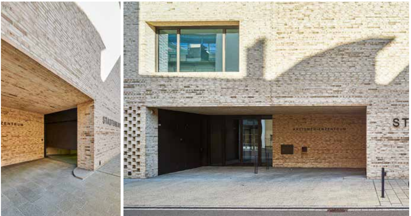
The exit of the underground car park is located on the longitudinal side of the building and is far less conspicuous than the entrance.
