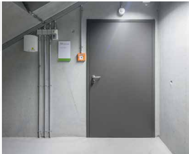
The door leaf fits flush with the profile frame.
