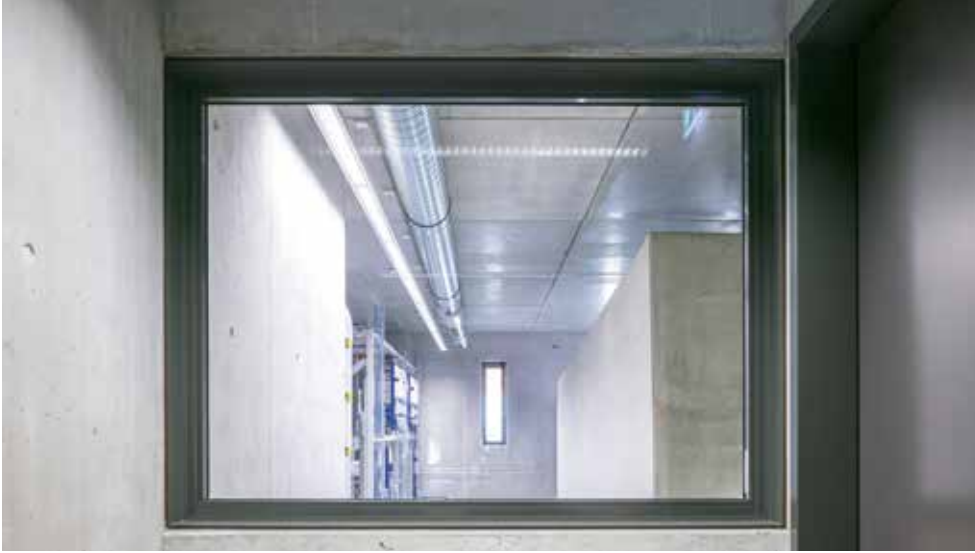
The end of the hallway provides a look into a room with a recessed building structure of unplastered concrete.
