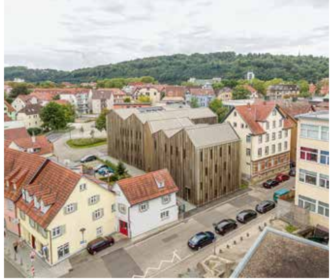
The facade of the institutional building is made up of anodised metal panels.
