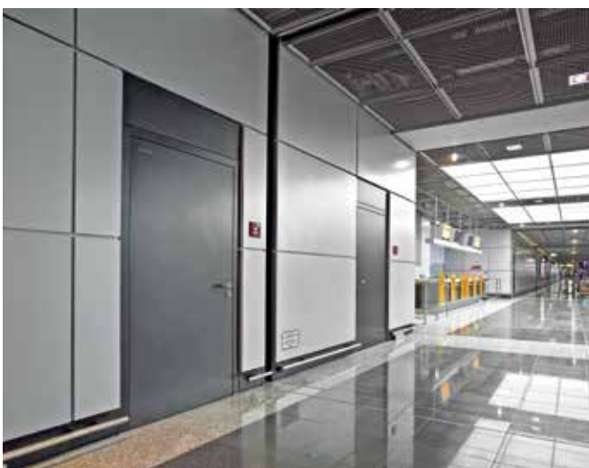
DryTec block frames are already backfilled with mineral wool.
