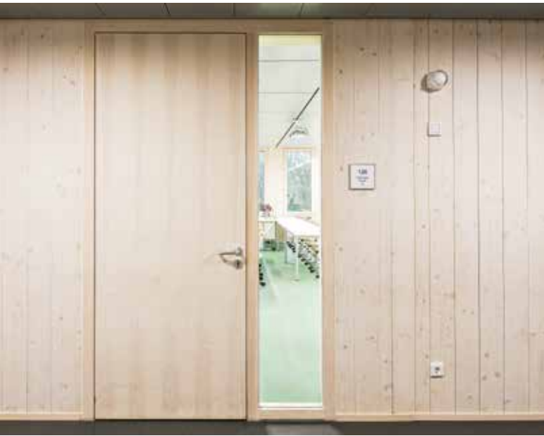
Fixed side elements allow passers-by to glance into the classrooms.
