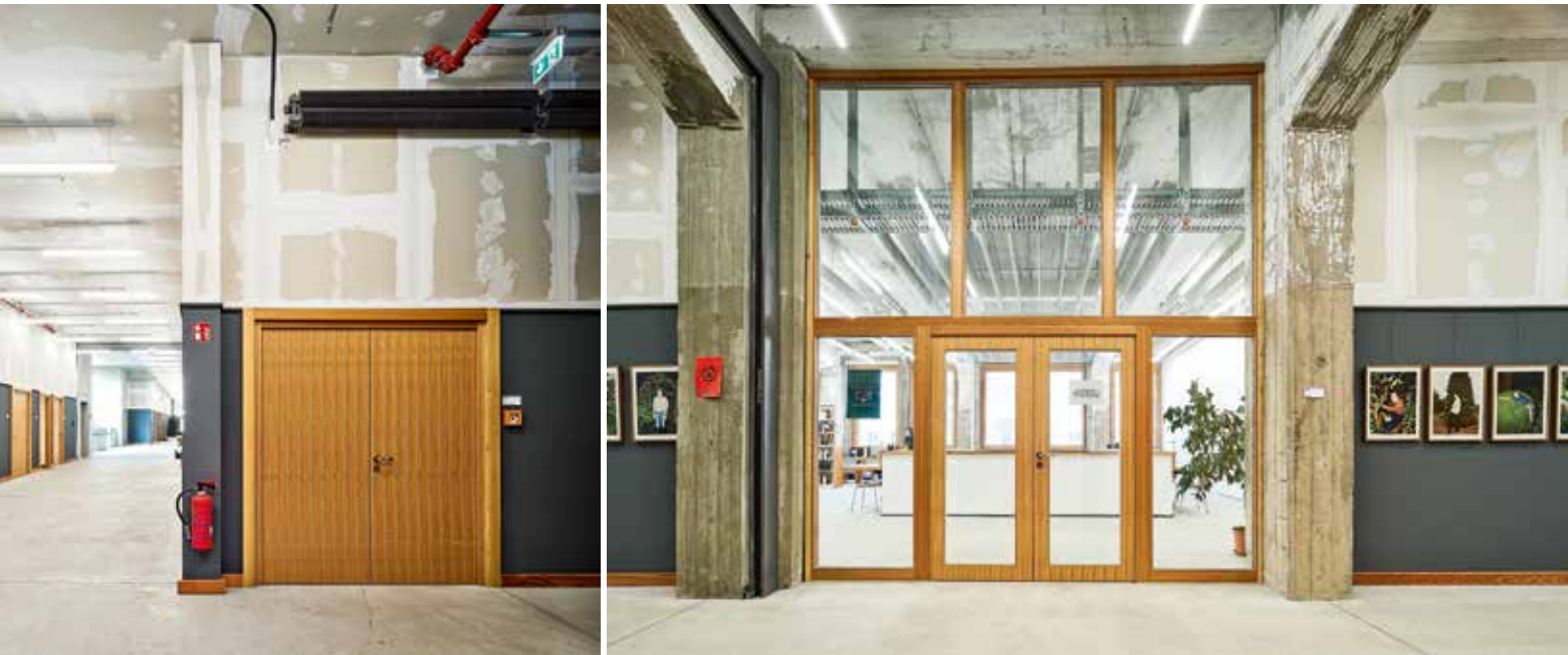
In terms of texture and colour, the larch wood forms a clear contrast to the raw walls as well as the anthracite-coloured wall cladding.
