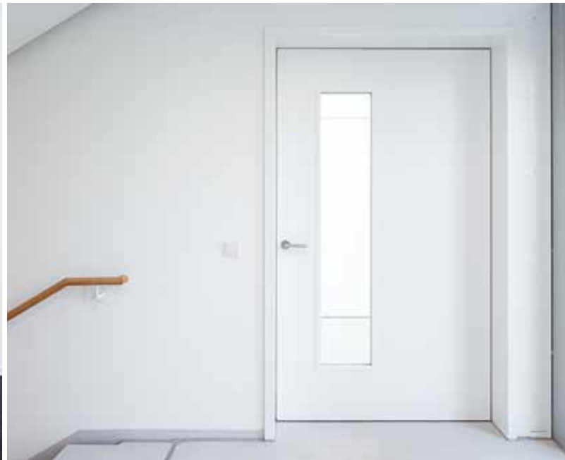
The fire-rated doors in the administrative area are in some cases solid (image left), while others feature a narrow glazing cut-out (image right).
