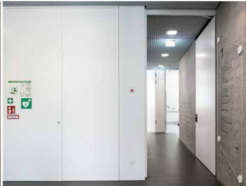
Normally open: the space-saving recess door.
