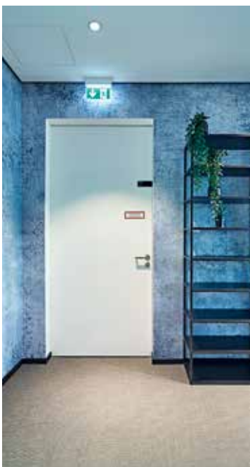
STS doors – fitted with block frames.
