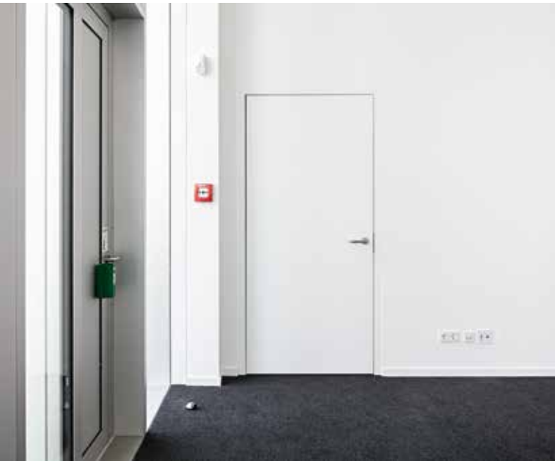
The fire-rated doors in the administrative area are in some cases solid (image left), while others feature a narrow glazing cut-out (image right).
