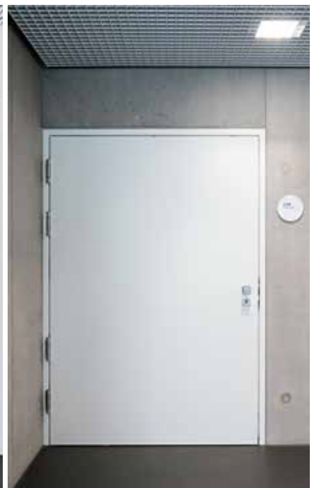
Several doors have excess width.
