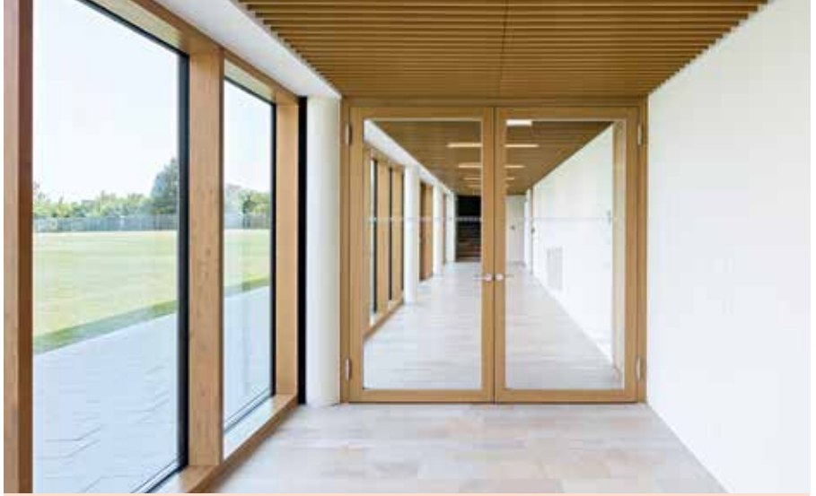
Sophisticated and generous: Seamless doors do not have a glazing bead.
