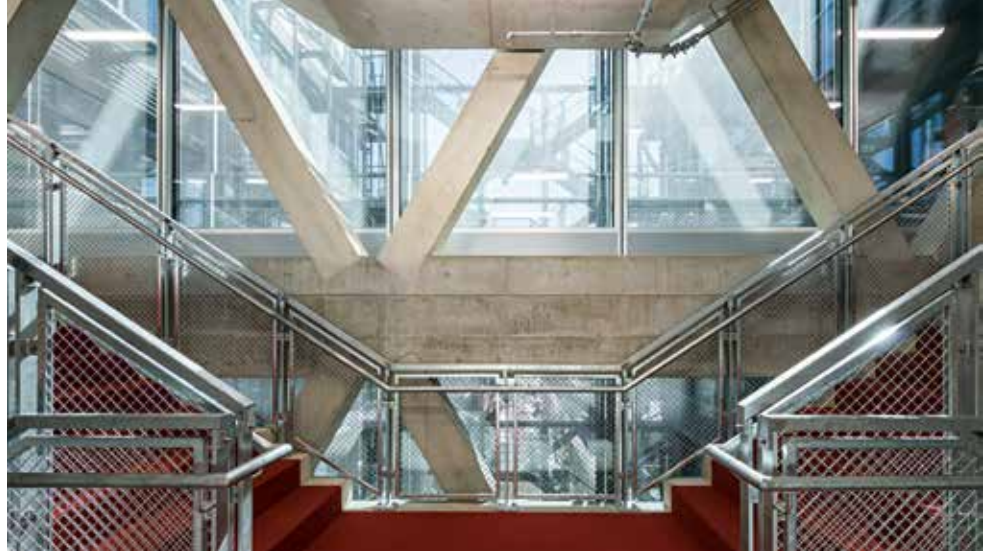
The raw support structure is visible everywhere in the building.
