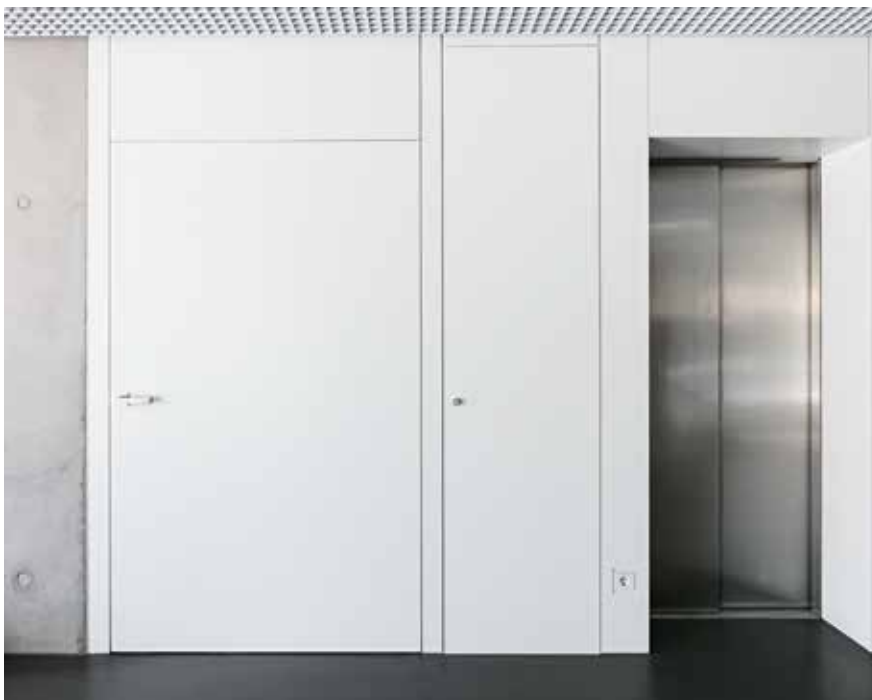
The doors with transom panel and solid timber block frame also fit the homogeneous overall look.
