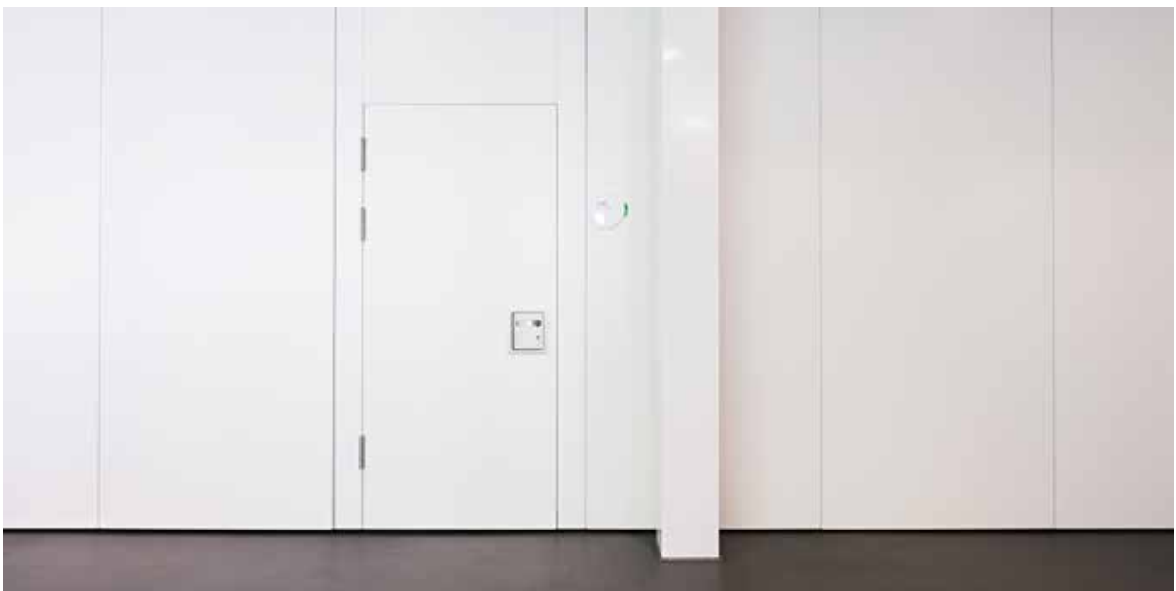
All doors are set flush in the wall.
