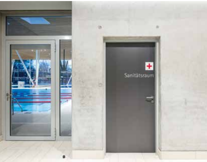
Most wet room doors are equipped with aluminium frames.
