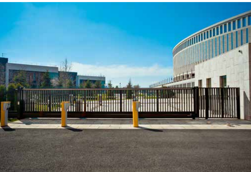
Only authorized persons may pass through the sliding gate.
