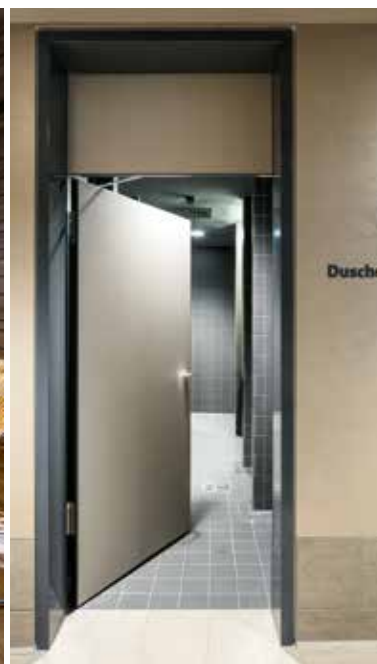
Wet room doors are manufactured free of wood and wood composite materials.
