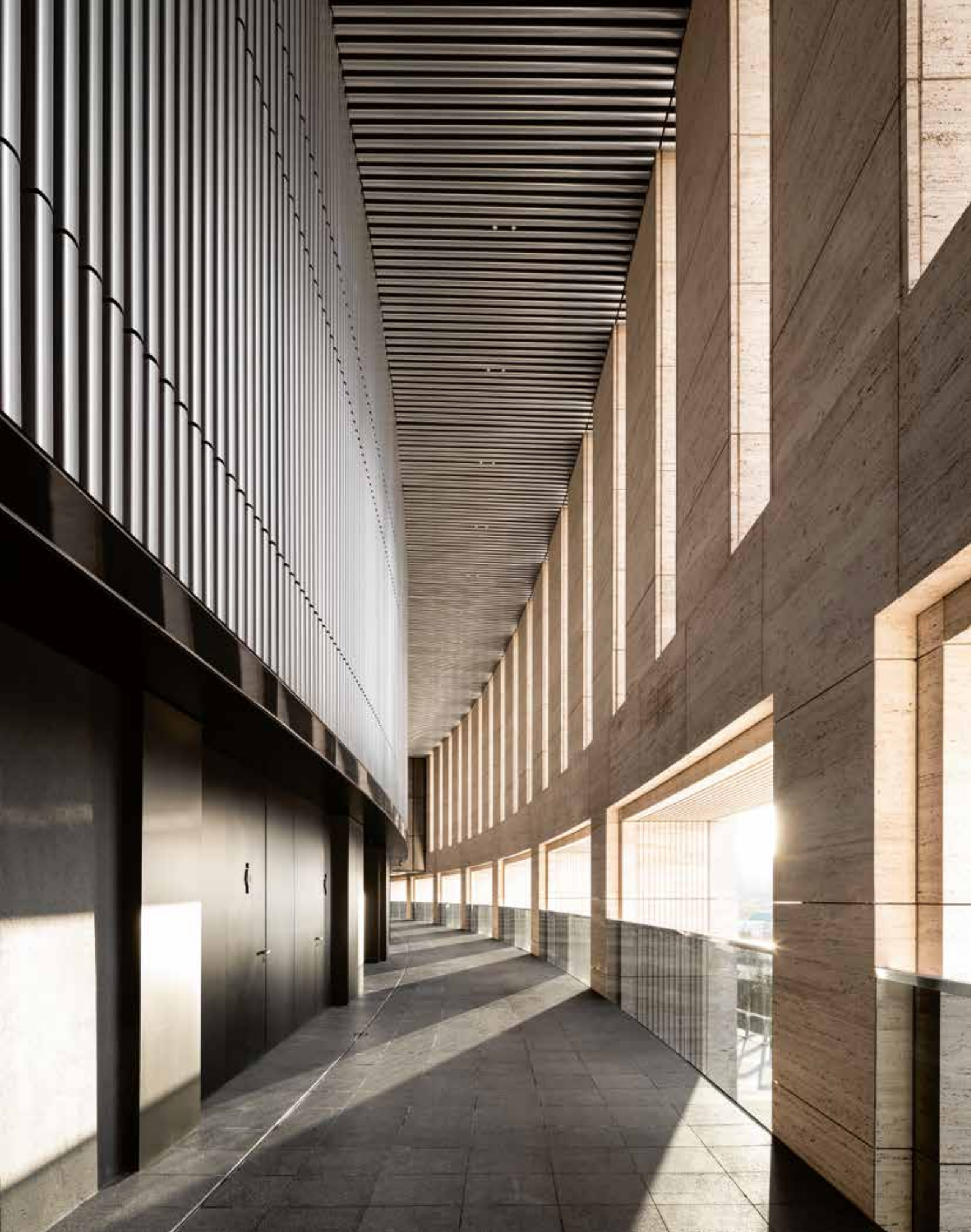
Noble choice of materials: Floor tiles made of black basalt and panels covered in anodised aluminium are rather infrequently found in stadiums.
