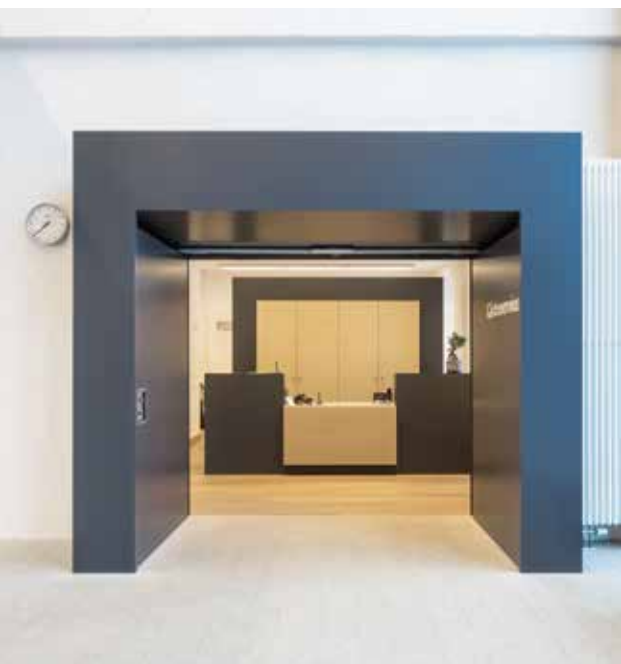
Recess doors allow barrier-free passage.
