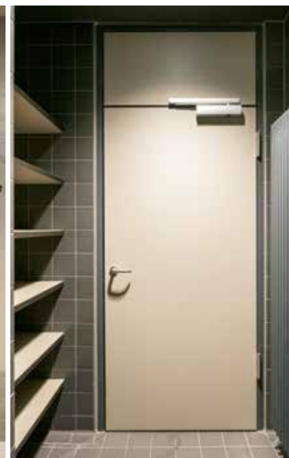
Wet room doors are manufactured free of wood and wood composite materials.
