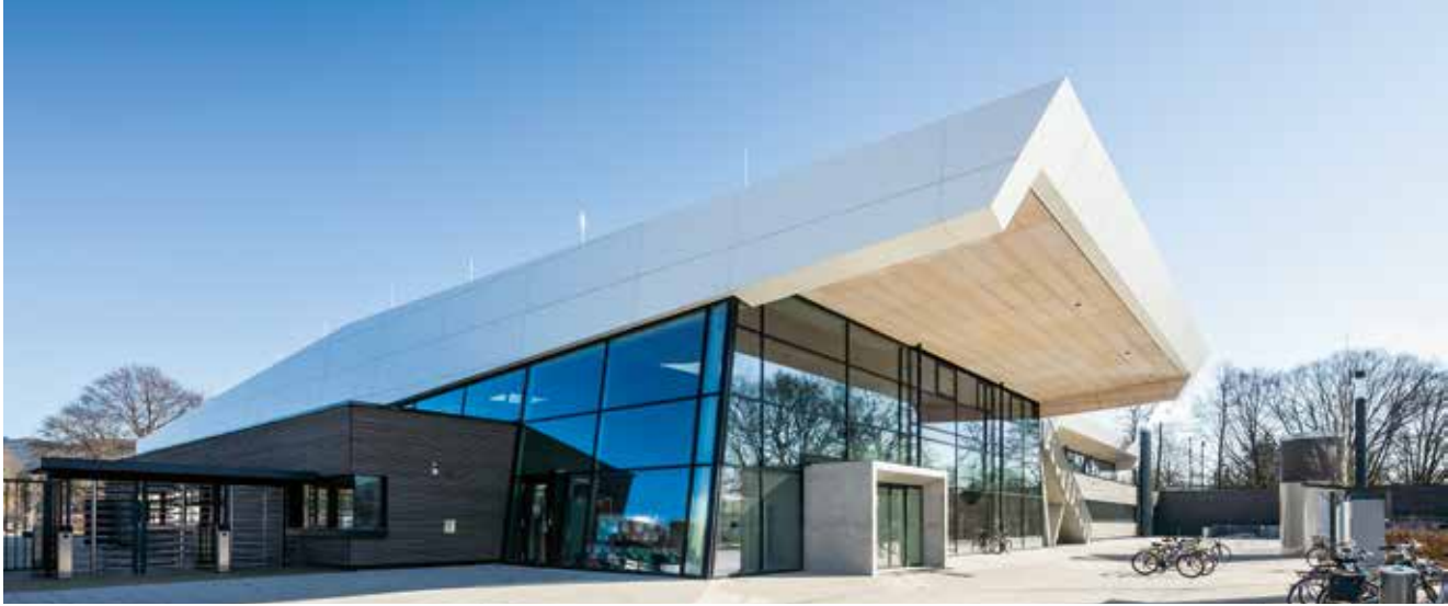
The expressive, widely projecting roof is the most dominant architectural feature of the building body.
