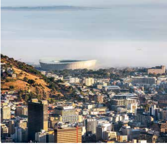
The Cape Town Stadium can accommodate a total of 68,000 spectators.
