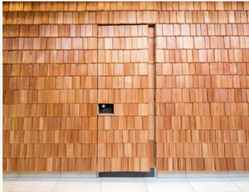
The doors were elaborately clad to integrate them into the wall.
