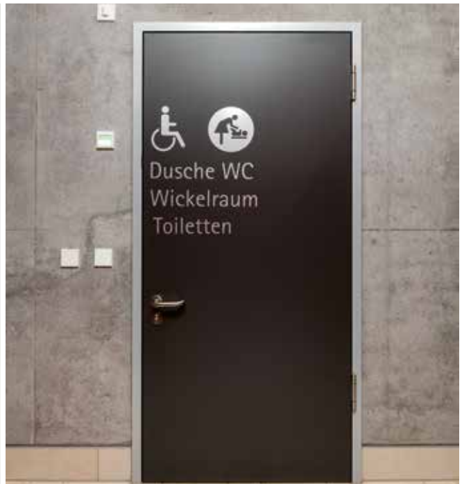
Frames in contrasting colours frame the barrier-free doors.
