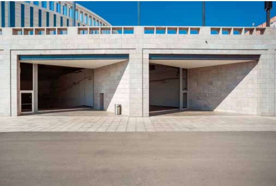
The access to the underground garage is closed by rolling grilles.
