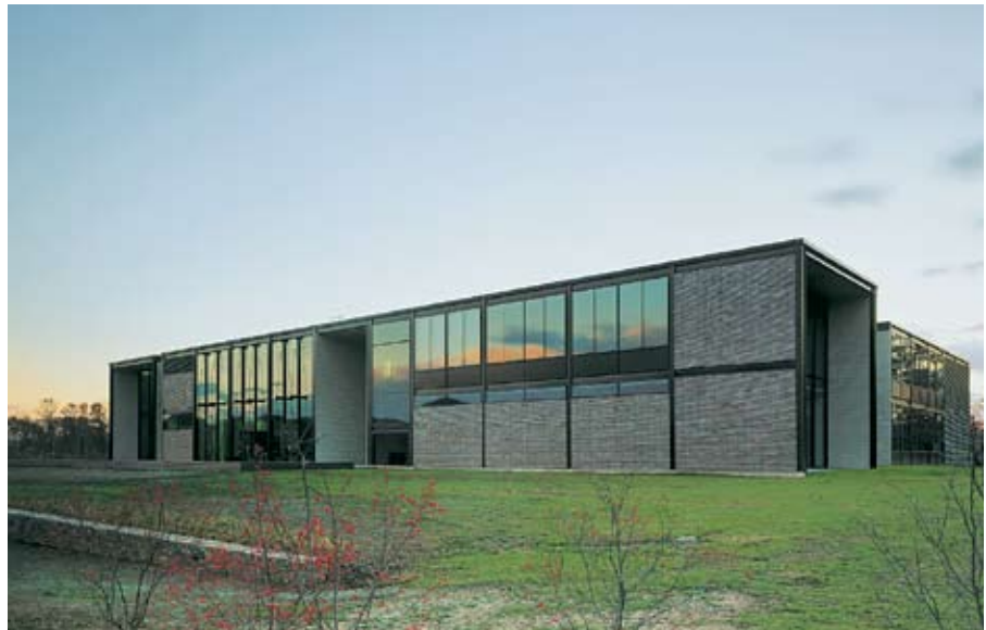
Customer and Training Centre in Farmington/Connecticut, USA (below). Business Incubator, Research and Administrative Building in Grünsch, Switzerland (far bottom).
